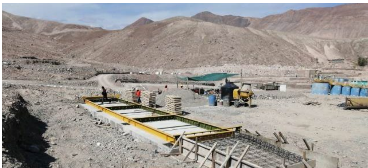
Figure 1: Installation of weighbridge (scales) at Cerro Dorado Site, Arequipa, Peru, November, 2019.
